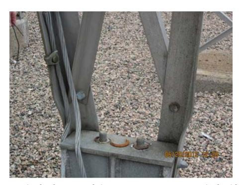
Figure 3: Example of Deformation of Aluminum Structure Legs as Result of Uplift Stresses
