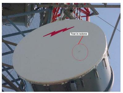
Figure 2: Tear in Radome
