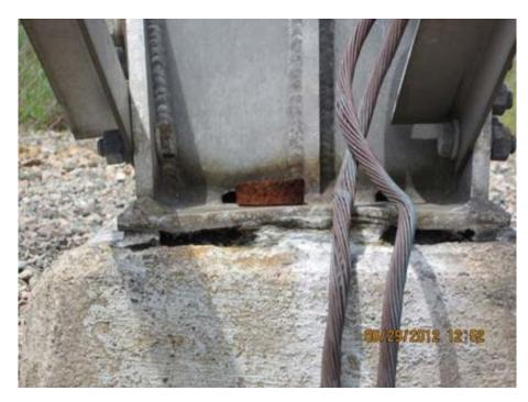
Figure 2: Example of Deformation of Baseplate Due to Aluminum Oxide Uplift
