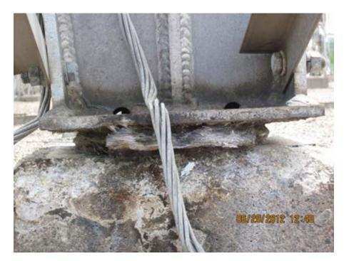
Figure 1: Example of Aluminum Oxide Formation between Concrete Surface and Aluminum Baseplate
