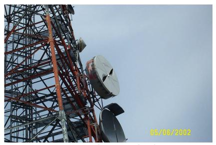
**Figure 3: Heavily Damaged Radome**
